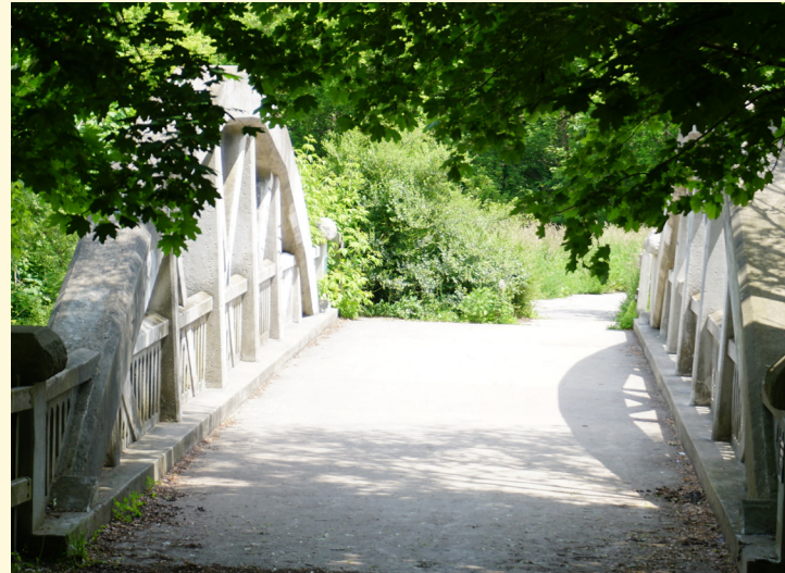
Middle Road Bridge
